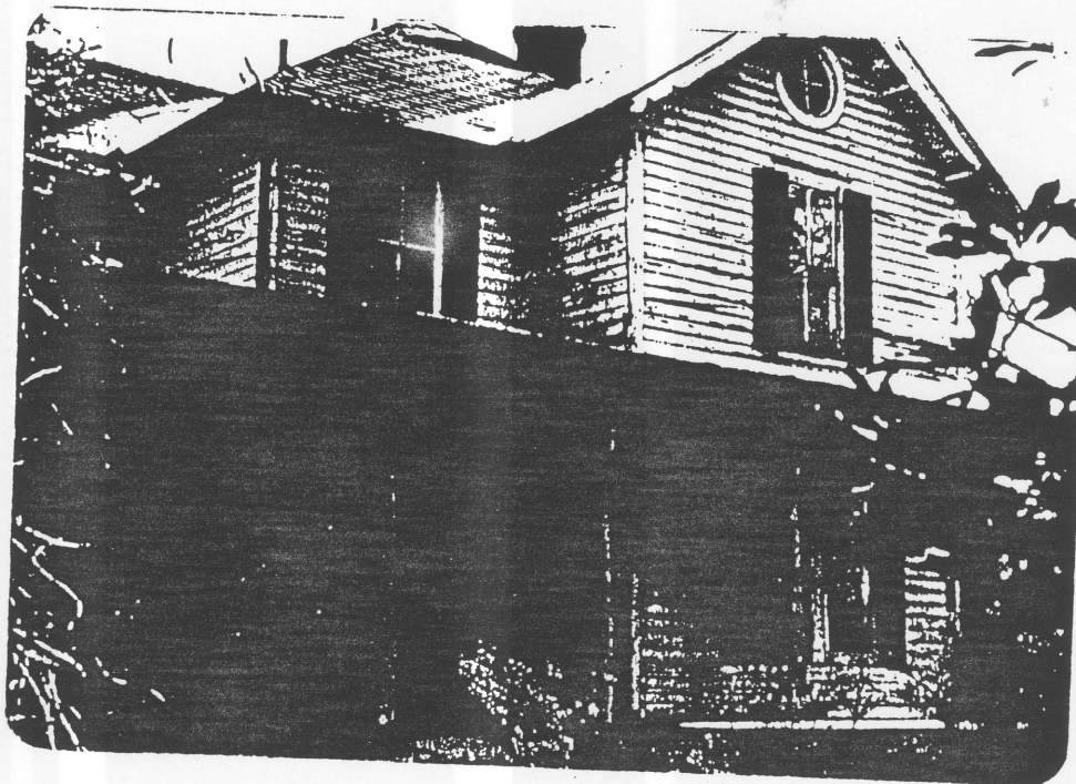
Front View Kolb-Bridges-Payne House 133 S. Pershing Drive
