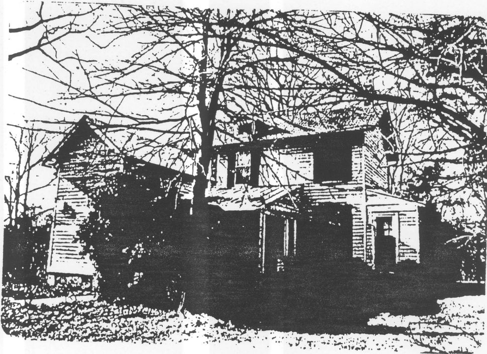
Back View Kolb-Bridges-Payne House 133 S. Pershing Drive Called "Woodmeade" by the Kolbs and "Mocking Bird Hill" by Mrs. M.B. Payne
